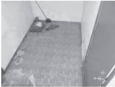
mud room behind garage
