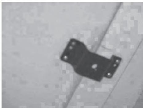
attic sealed shut/screws
